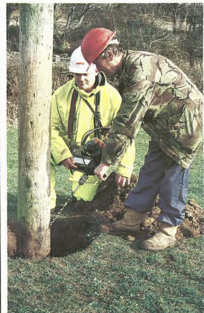
Manweb is in the process of treating all its poles with borate preservative to extend the life of what is a valuable network asset. Here Alf Parry (right) from UTEC is preparing a pole while Manweb linesman Chris Powell gets to grips with the Hunter hand held computer.
